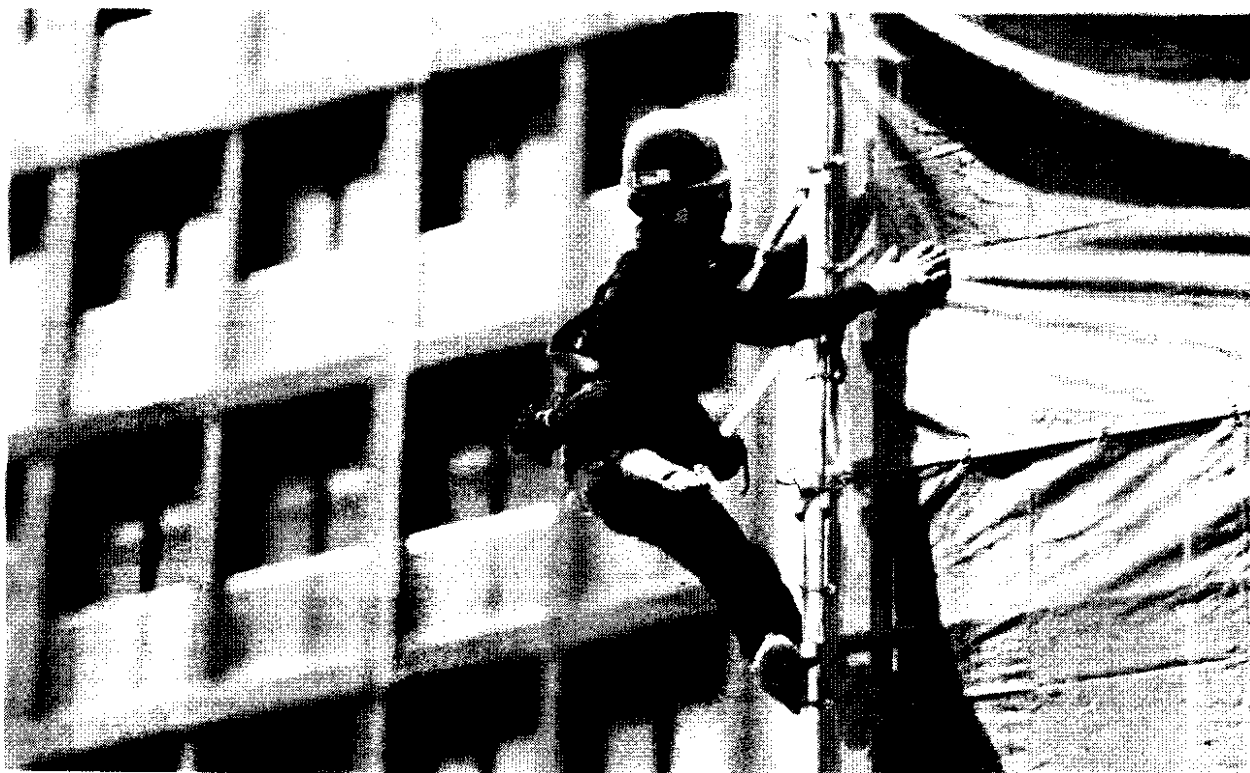
A man works at a construction site on Phloenchit Road in Bangkok. The government is budgeting for a larger deficit in fiscal 2018 to boost the economy as private investment remains tepid. SEKSAN ROJJANAMETAKUN
