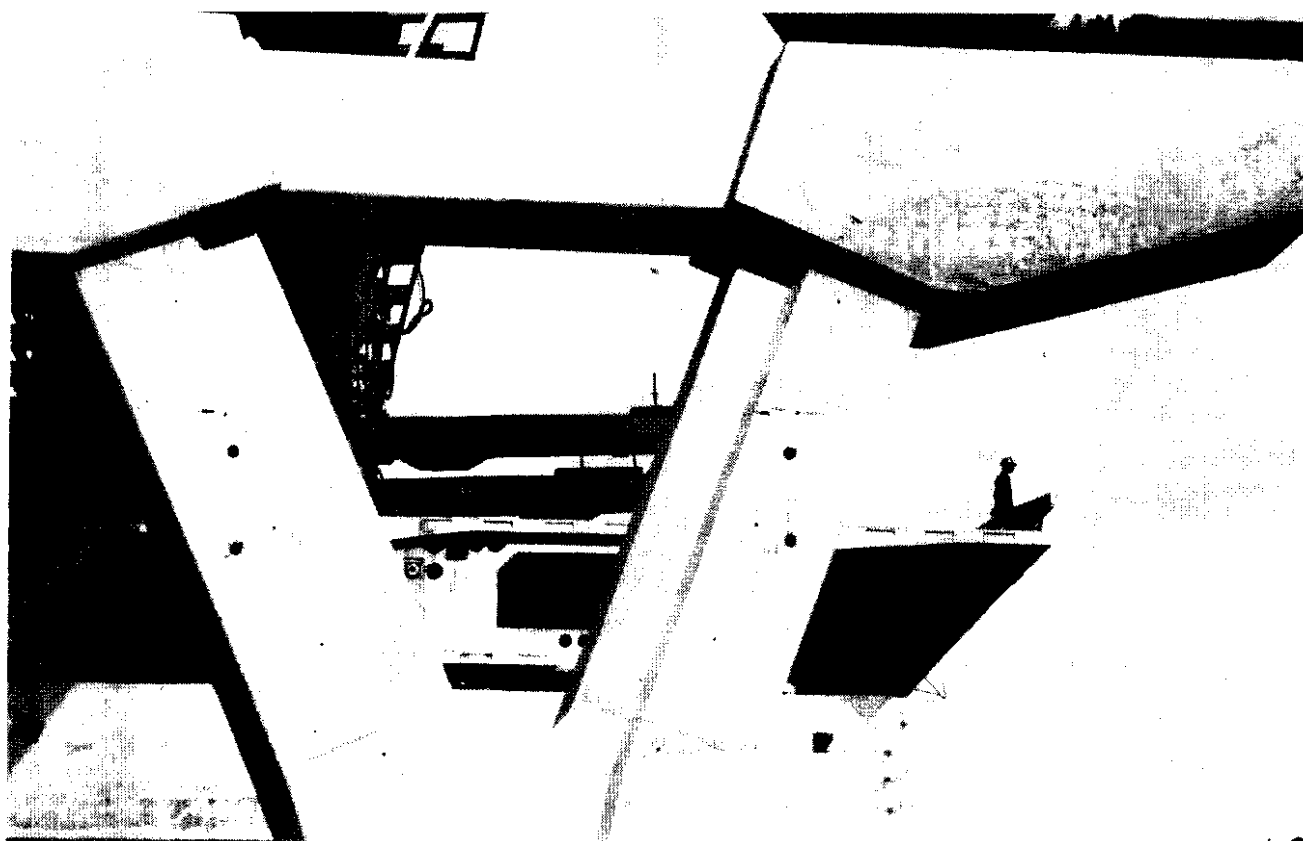
A worker stands at an expressway construction site in Bangkok's Bang Sue district. Infrastructure investments are likely to play a key role in driving the economy this year. PATTARAPONG CHATPATTARASILL 19
