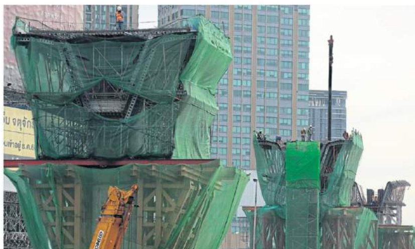
Workers construct supports for the skytrain's Mor Chit-Saphan Mai-Khu Khot section. To reach 4% full-year growth, GDP will likely have to expand 4.7% in Q4. PATIPAT JANTHONG
