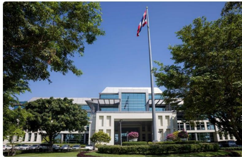
The Bank of Thailand complex in Bangkok. (Photo: Bloomberg)
