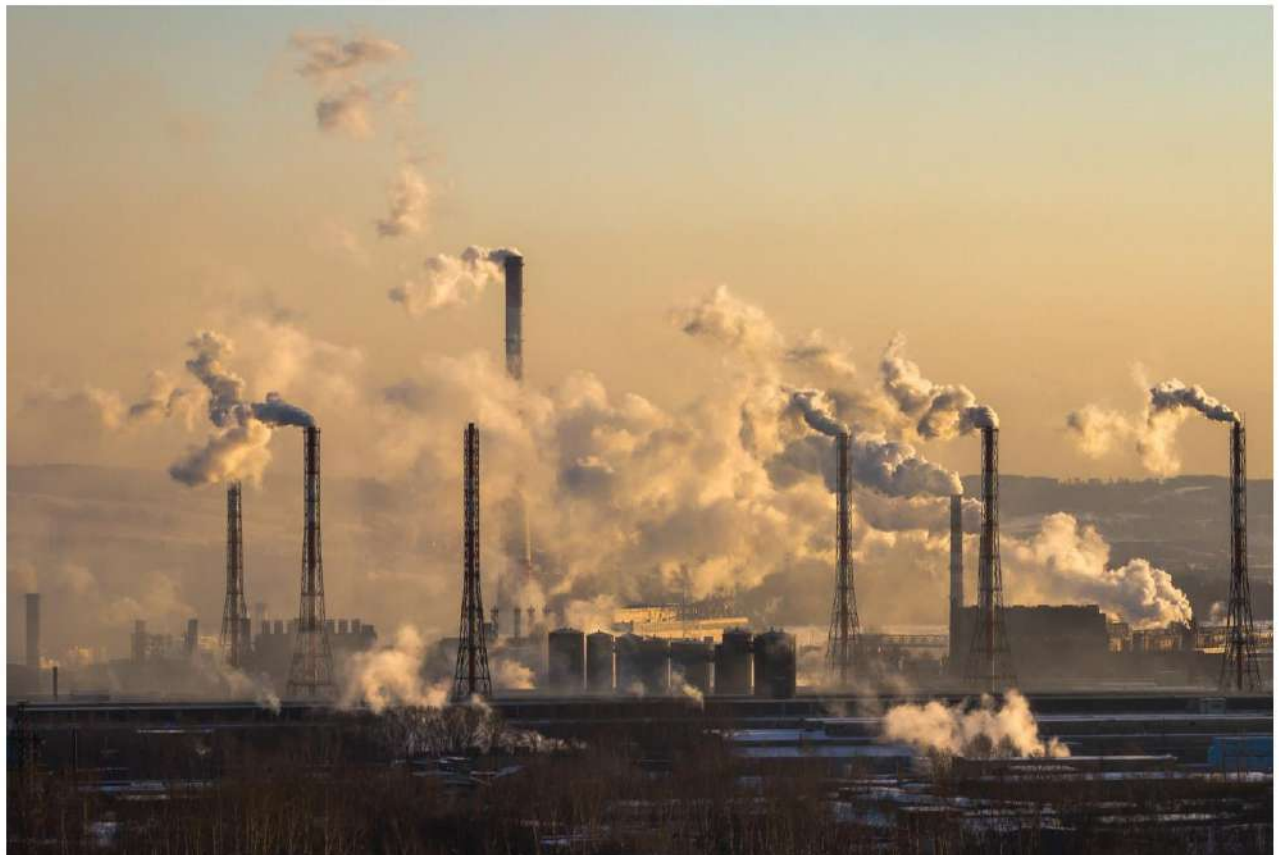
Emissions are emitted from chimneys at an industrial plant. The Excise Department is proposing a ministerial regulation for carbon tax collection, which has already been endorsed by the Finance Ministry.
