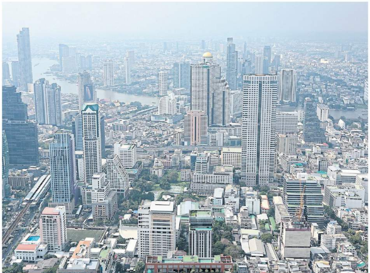
An aerial view of buildings in Bangkok. Mr Paopoom says the proposed improvements to the land and building tax aim to enhance both efficiency of collection and levy an appropriate rate. PATIPAT JANTHONG
