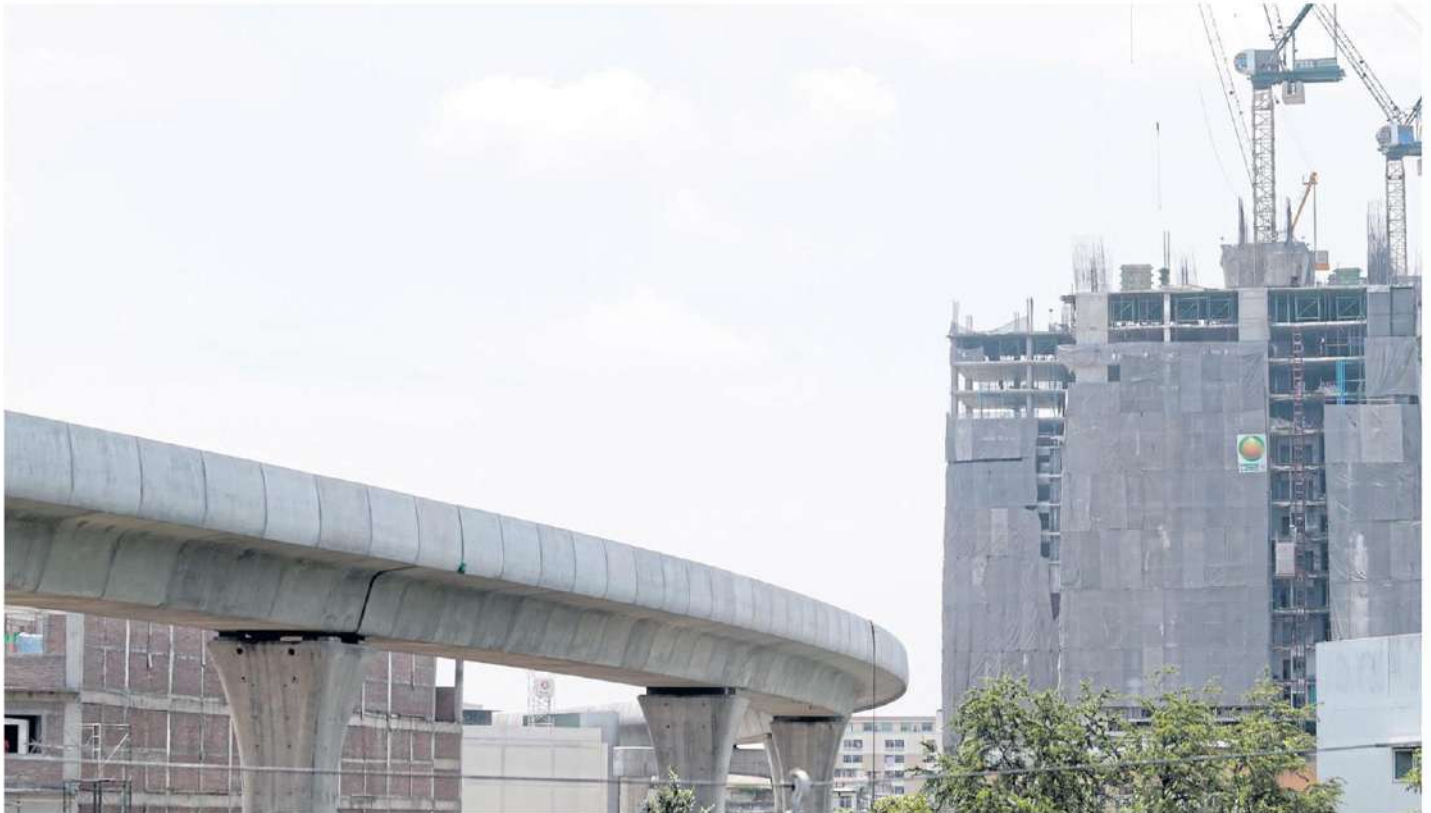
A condominium rises along an elevated mass transit project. PATTARAPONG CHATPATTARASIL
